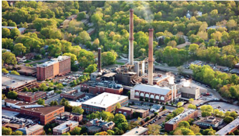
The University of Missouri's combined heat and power (CHP) plant is among the nation's leaders at producing green energy.
