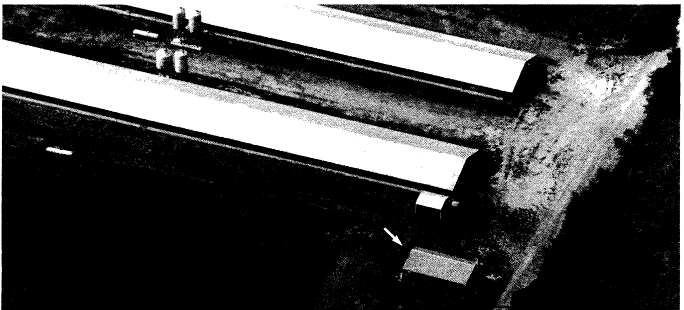
The Wallace broiler production facility with composter. Composters should be positioned close to the buildings for ease of accessibility
