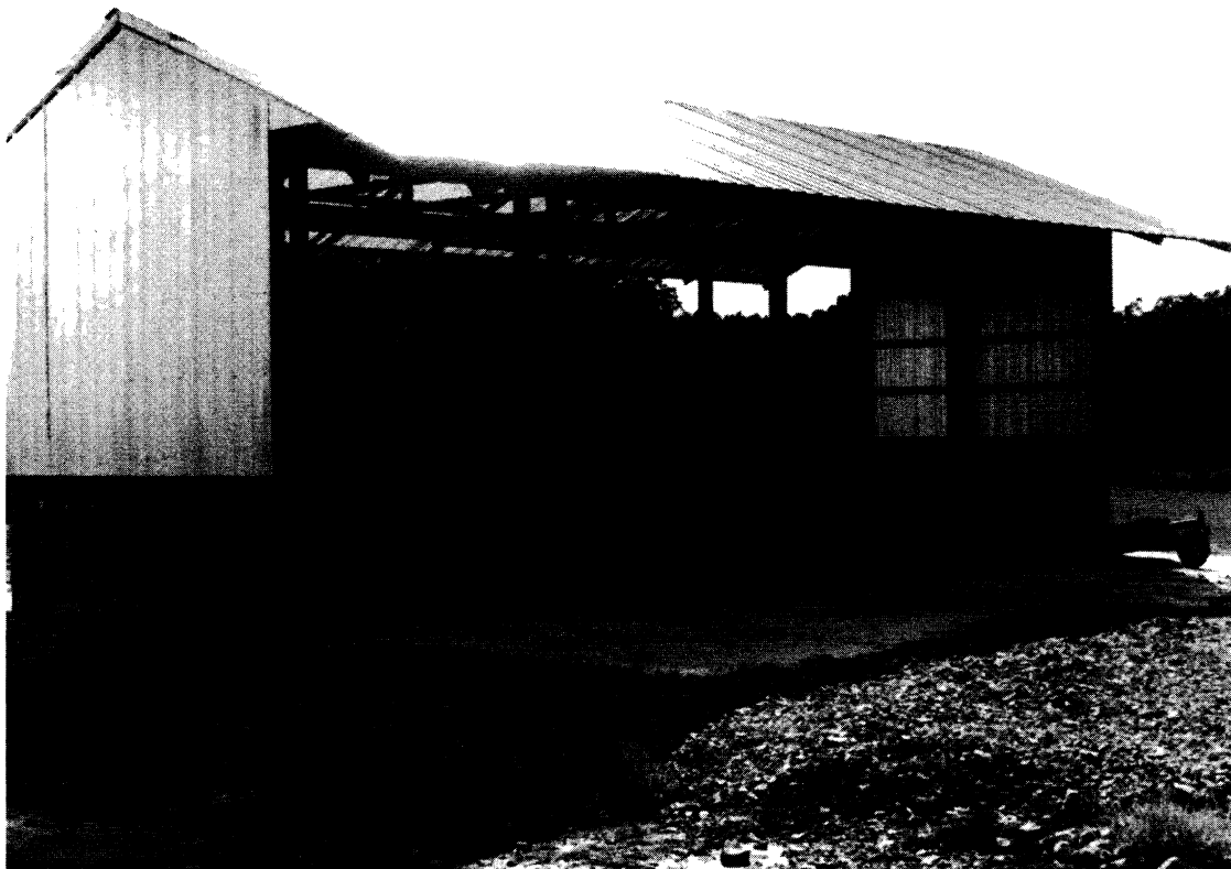
"Umbrella" type construction allows access to composting bins from either side of the Harvill composter.
