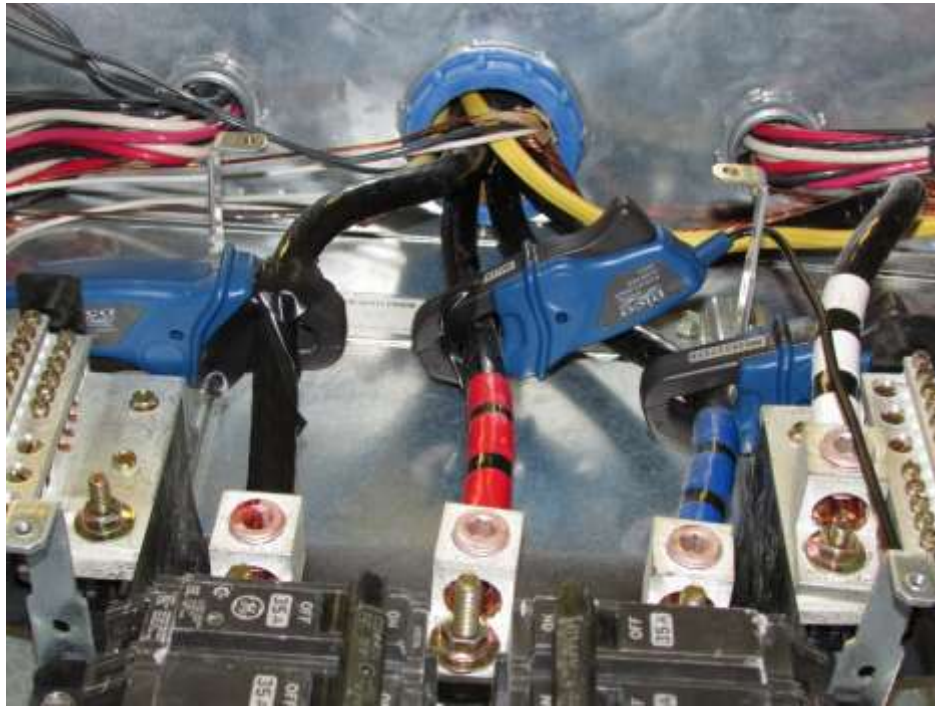
Figure 14 Current Clamps Installed inside the Circuit Breaker
