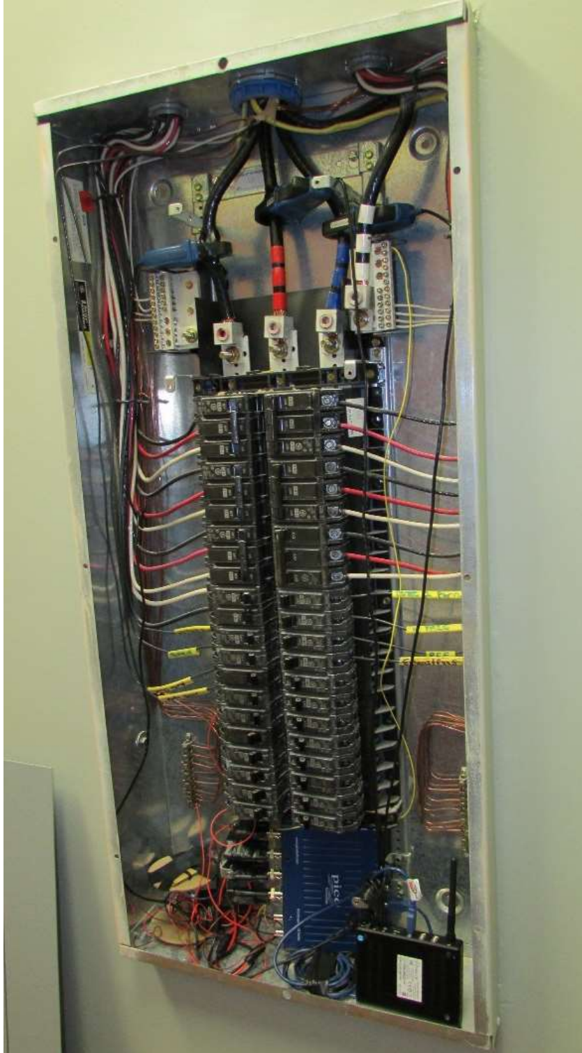
Figure 24 NILM wireless data Acquisition installed inside the circuit breaker
