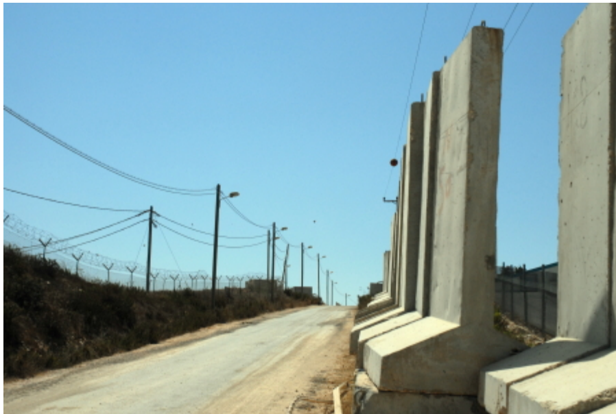
Figure 2-6 - Massive concrete walls provide shielding from blast loads and debris.
