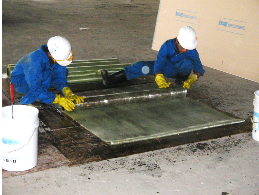
Figure 2-7 - Workers apply wet lay-up glass fiber reinforced polymer (GFRP) to a concrete slab. A large quantity of fabric can be easily shipped and stored, as it rolls compactly onto spools. (Fyfe 2012)
