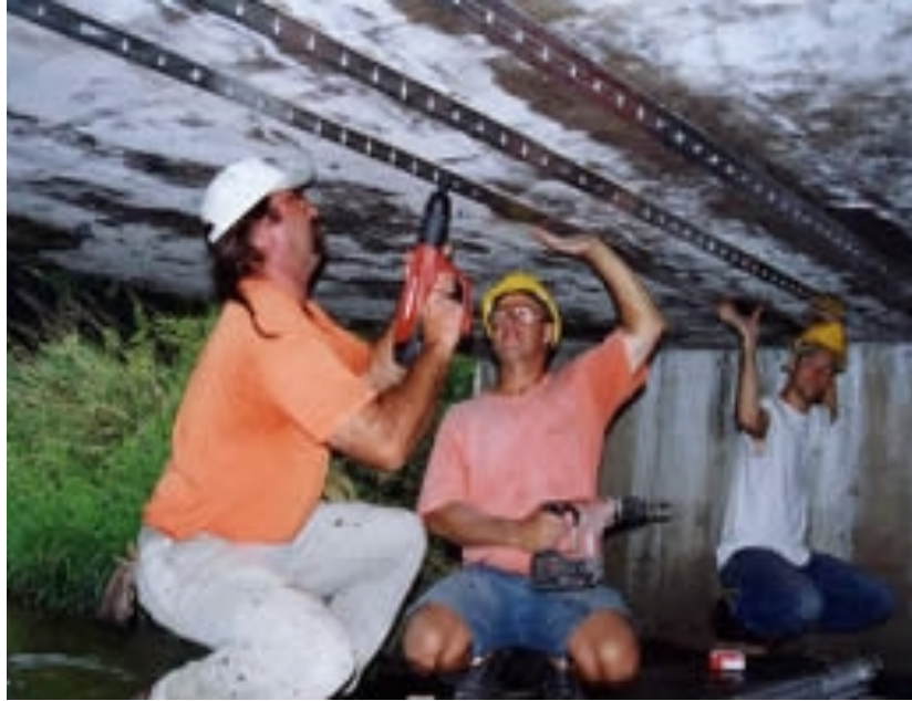
Figure 2-12 - Workers install pultruded FRP with mechanical anchors (Strongwell 2006).
