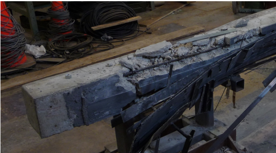
Figure 5-8 - Most of the concrete cover was sloughed off, and the CFRP completely delaminated.
