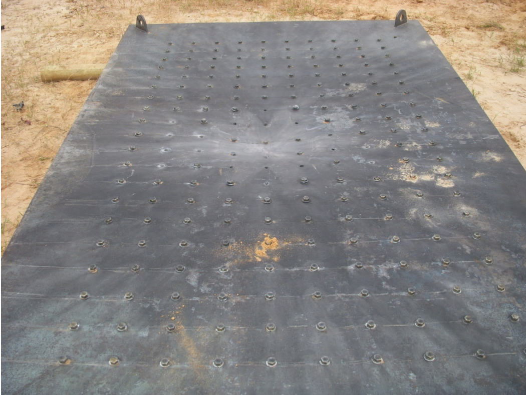
Figure 3-3 – Damage effects from a past blast test of a concrete slab with steel cladding on both faces through-bolted. Some bolt heads were sheared off, but the slab was not breached and the concrete was confined.
