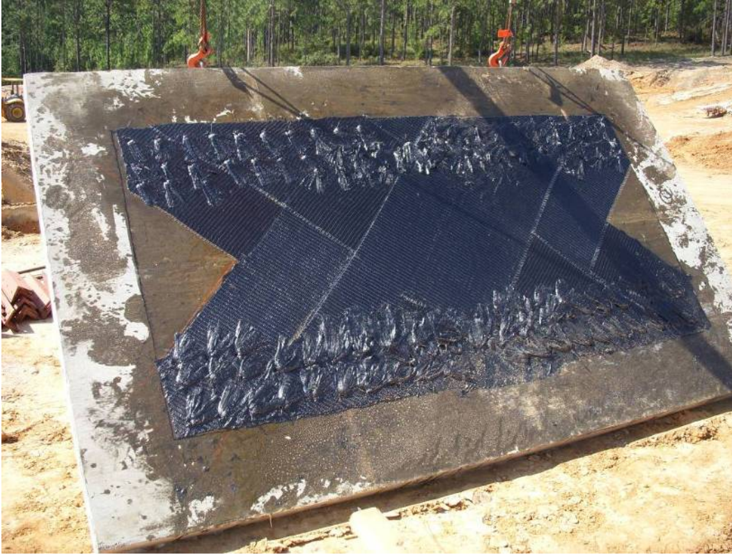
Figure 2-21 - Wet-layup CFRP applied to the tension face of a concrete slab to be tested at a scaled range of 1.5. Note the extensive use of fiber anchors (Orton 2013).
