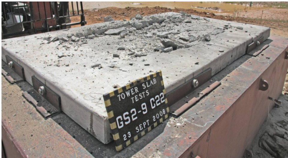
Figure 2-22 - Wet-layup CFRP strengthened slab tested at scaled range 1.5, post-test. The slab did not breach.
