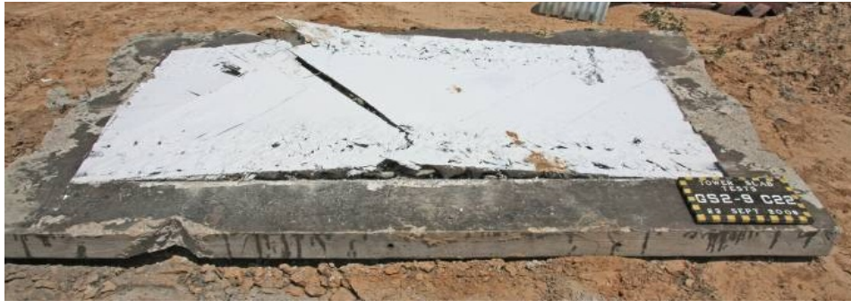
Figure 2-23 Wet-layup CFRP strengthened slab tested at scaled range 1.5, post-test, reverse side. Though the CFRP fractured, the slab did not breach.
