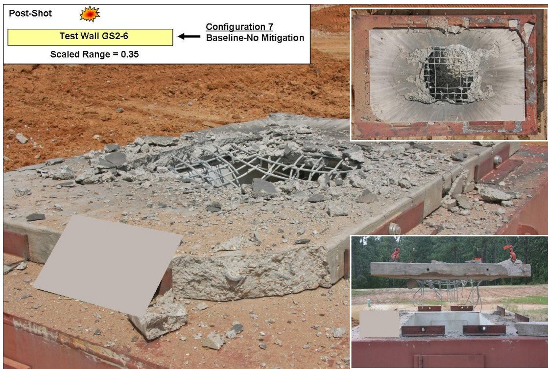
Figure 3-1 – Damage experienced in a past blast test of an un-mitigated concrete slab at 0.35 \text{ ft/lb}^{1/3} scaled range. Slab was exposed to a peak pressure over 50,000 psi and catastrophic breaching of the slab occurred (Ray et al. 2011).
