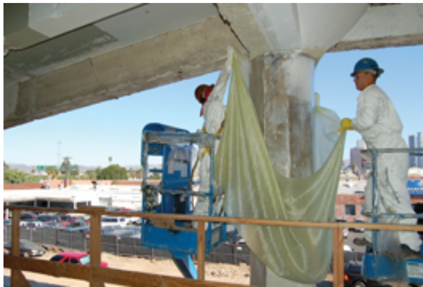
Figure 2-10 - Workers install wet-layup glass fiber reinforced polymer (GFRP) on a reinforced concrete column (Fyfe 2012).
