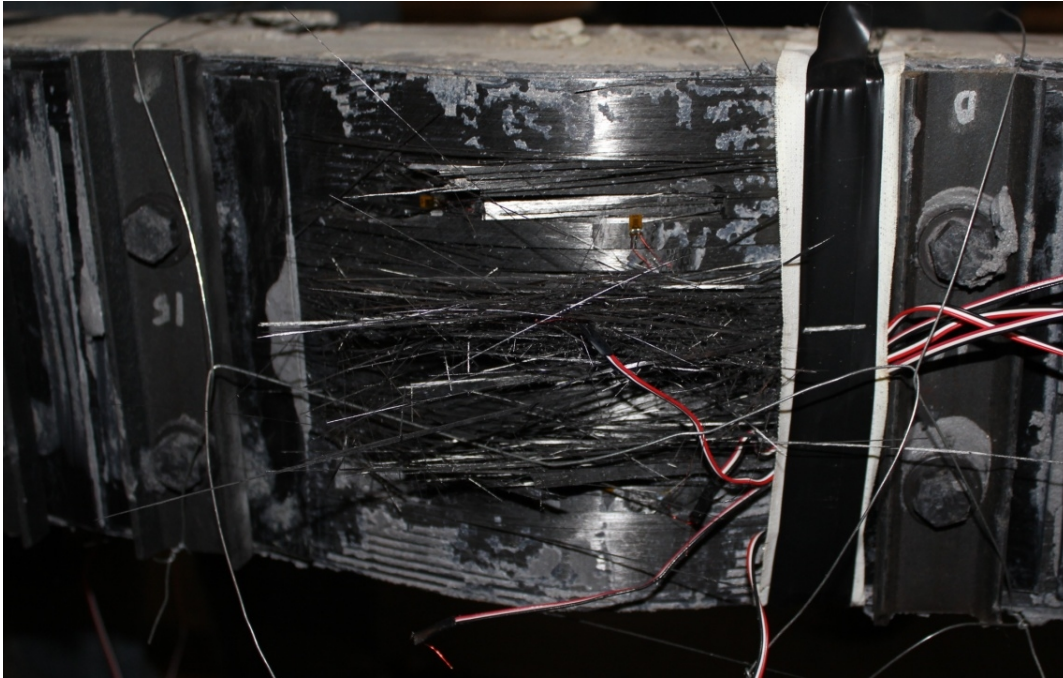
Figure 5-6 - Much of the longitudinal FRP at midspan was fractured, despite slipping and splitting.
