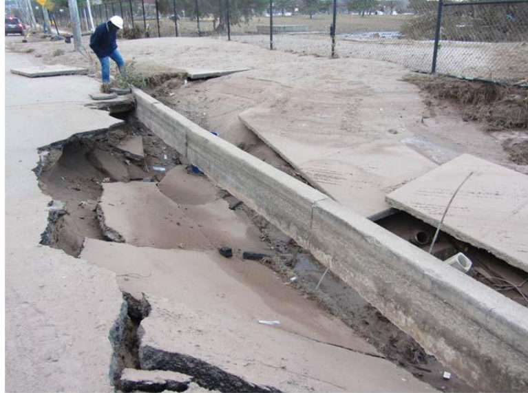
Figure 1.8 Damage due to scouring on street, curb, sidewalk and utilities, [10]
