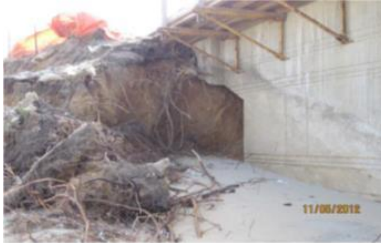
Figure 1.3 Erosion at the southeast abutment wall [10]
