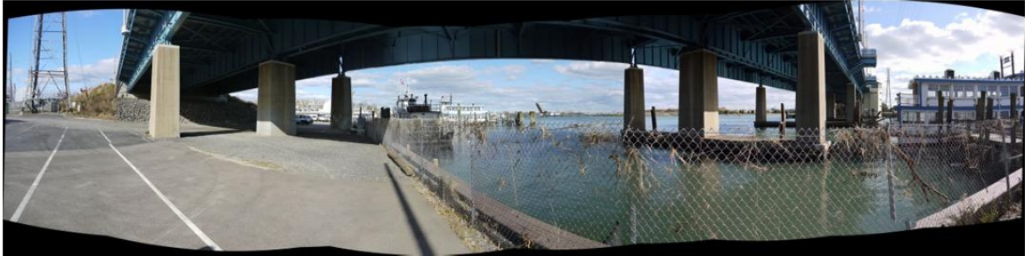
Figure 1.5 North abutment of route 35 Draw Bridge over Manasquan River, [10]
