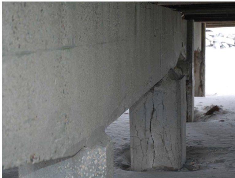
Figure 1.7 Scouring and cracking observed in concrete piers, [10]
