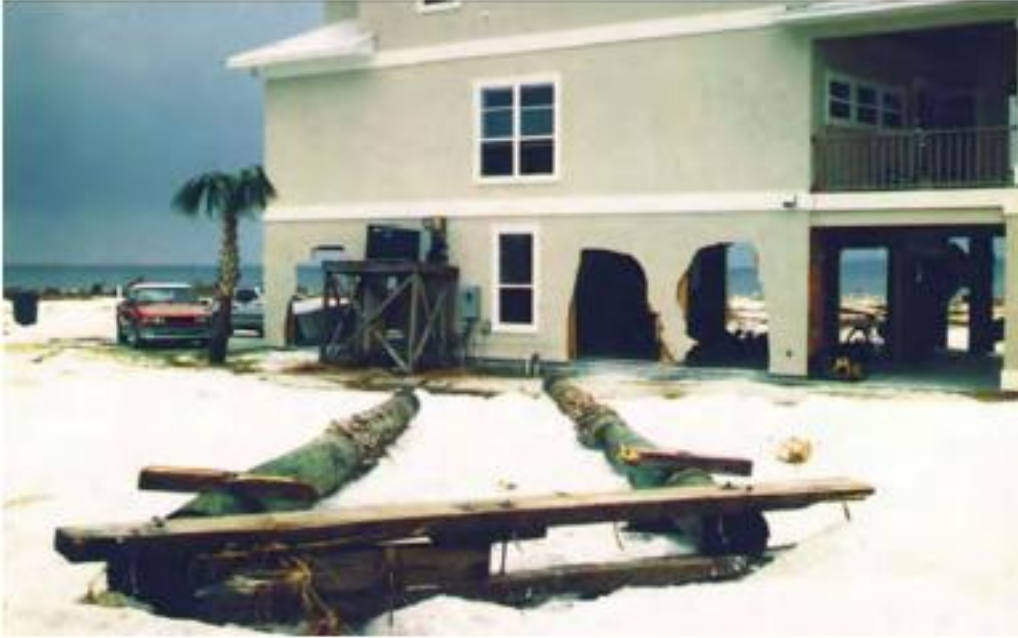
Figure 2.2 Damage as a result of debris impact [12]
