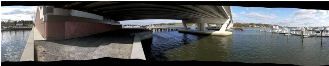
Figure 1.6 Route 70 bridges over the Manasquan River, [10]
