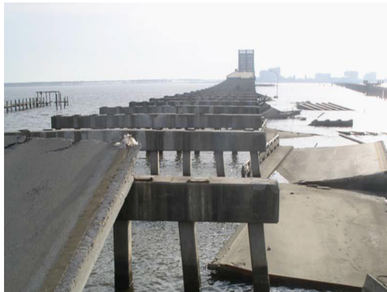
Figure 1.2 Span unseating due to storm surge induced loading for US- 90 Biloxi Bridge [7]
