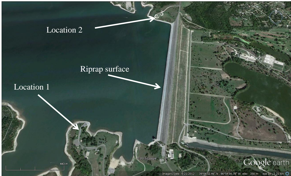
Figure 5.2 Google earth image of Milford Dam showing radar locations relative to dam structures.
