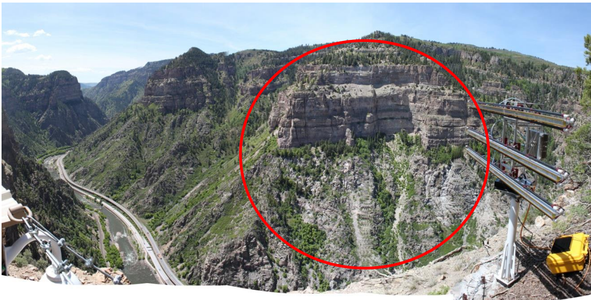
Figure 4.4 Panoramic view from radar location. Red circle indicates primary site of interest.
