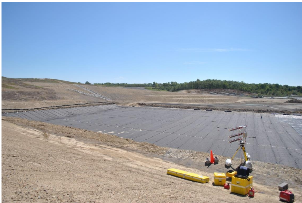
Figure 6.2 Looking onto the site of interest (Cell 5) from Cell 4. The black surfaces are areas of the compacted clay liner overlain with geosynthetic material
