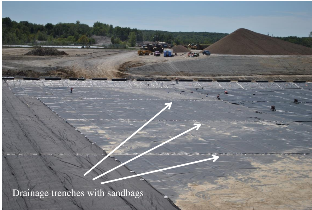
Figure 6.6 Zoomed-in view of geosynthetic liner, showing drainage trenches with sandbags in the trenches restraining movement of the liner.
