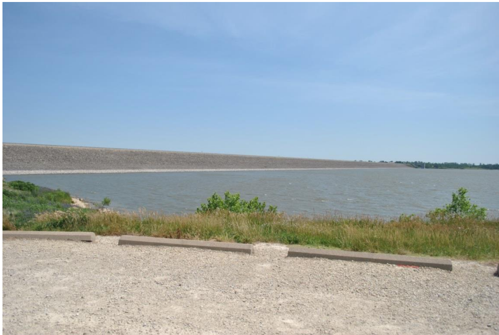
Figure 5.3 Photograph of Milford Dam taken from the vantage point of Location 2.
