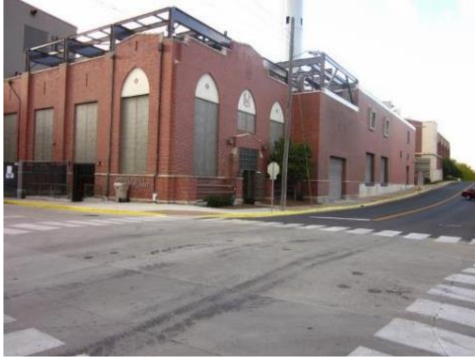
Figure 8: University of Missouri power plant, an unsafe area
