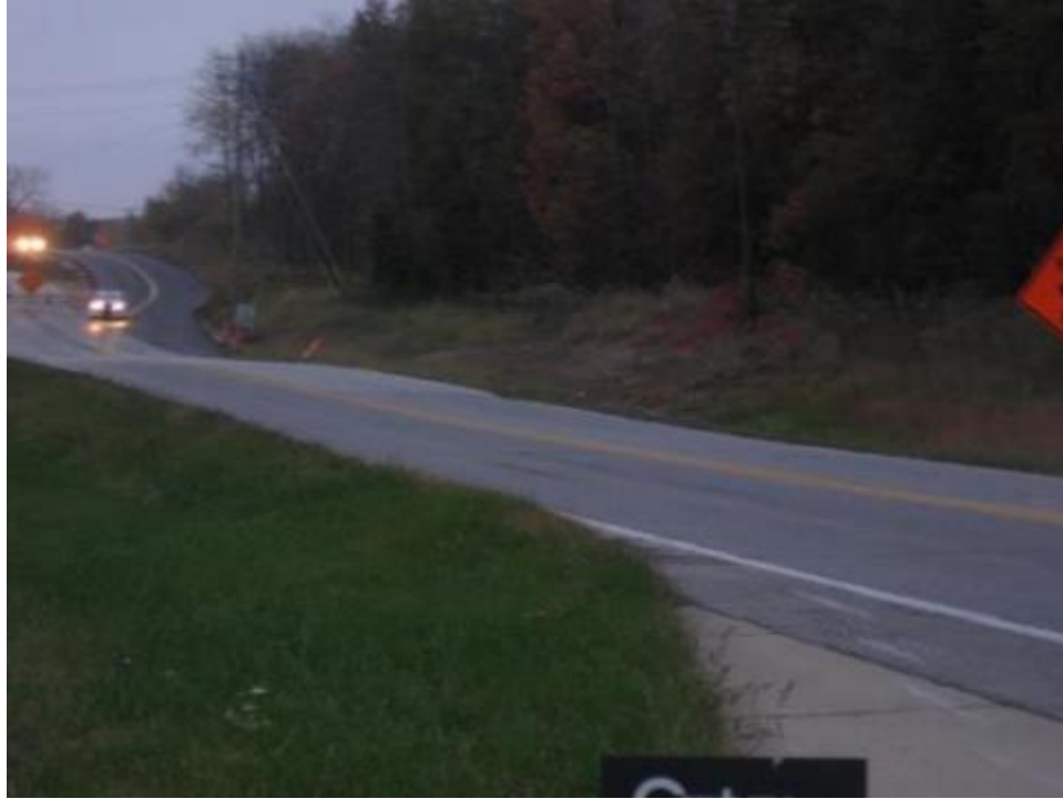
Figure 13: A dangerous bus stop with no sidewalk for pedestrians
