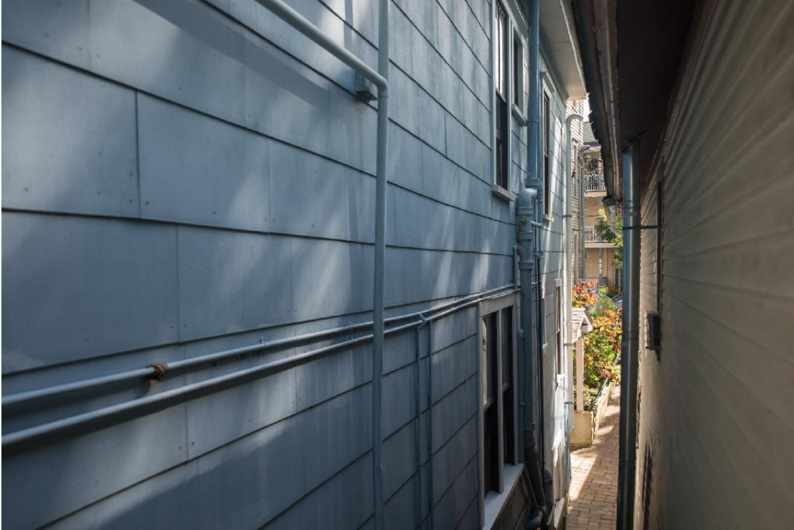
Fig. 7 A small alley in between houses
