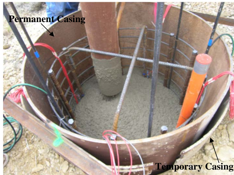
Figure 3.15- Drilled shaft with temporary and permanent casing. The temporary casing was removed following concrete placement.
