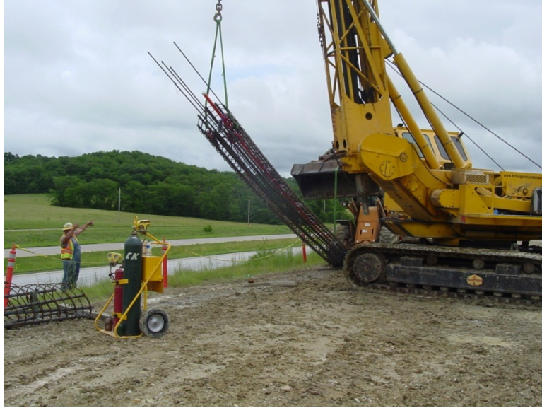
Figure 3.16 - Hoisting of reinforcing cage using the drilling rig at the top of the cage and front end loader at the O-cell™.
