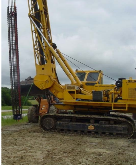
Figure 3.12- Watson-3100 CM rig used to construct test shafts at the Frankford Load Test Site.
