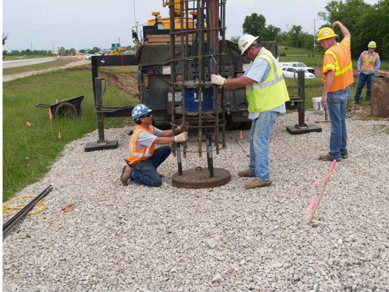
Figure 3.8 - Photograph of post-grouting plate being attached to the reinforcing cage prior to placement in the hole.
