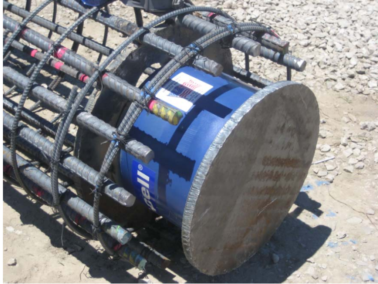
Figure 3.17 - Osterberg Cell™ attached to the base of a reinforcing cage.
