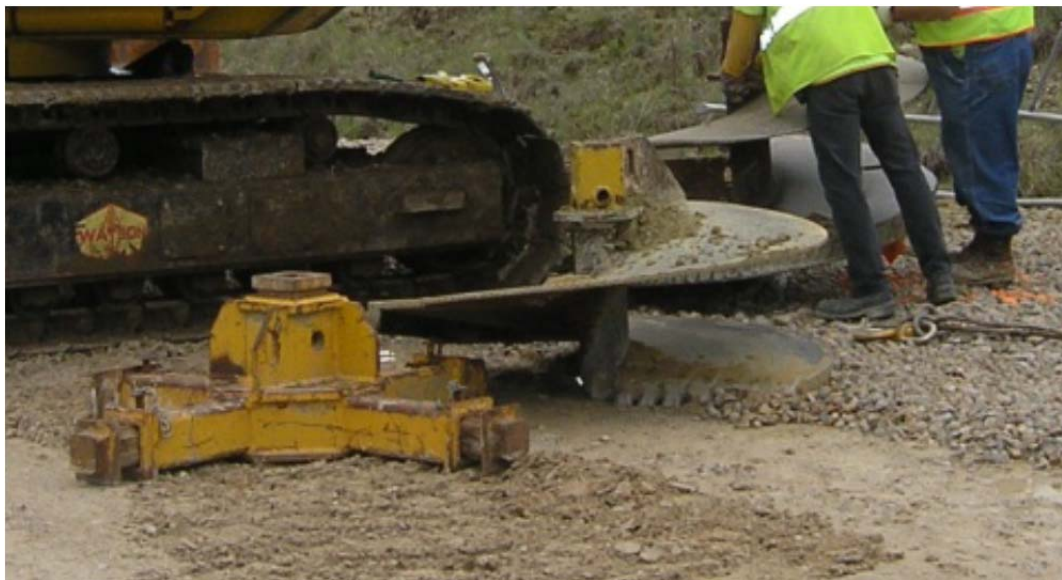
Figure 3.13- The 60-inch auger used to excavate 60-inch diameter shafts at the Frankford Load Test Site
