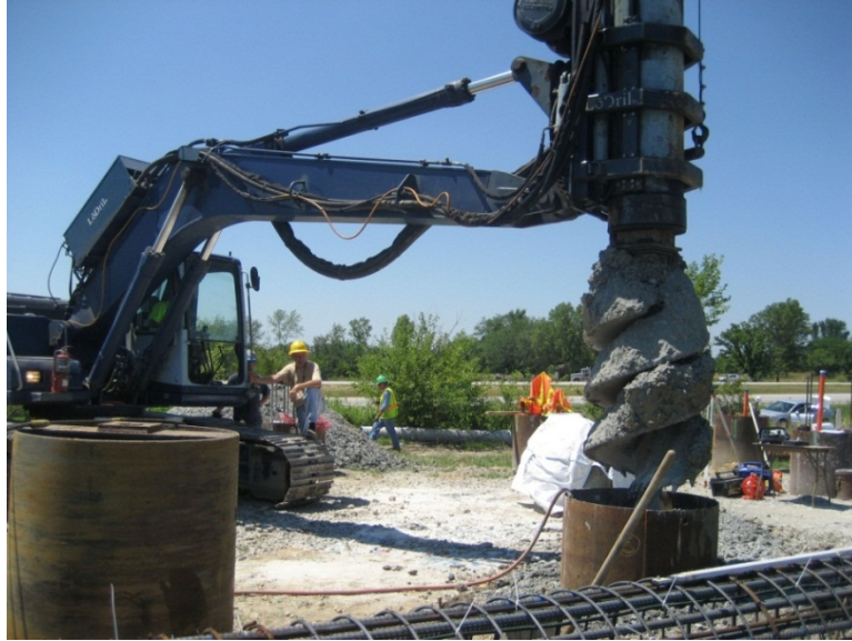
Figure 3.5- LoDrill (model number LLMHTFB50) rig used at the Warrensburg Load Test Site.
