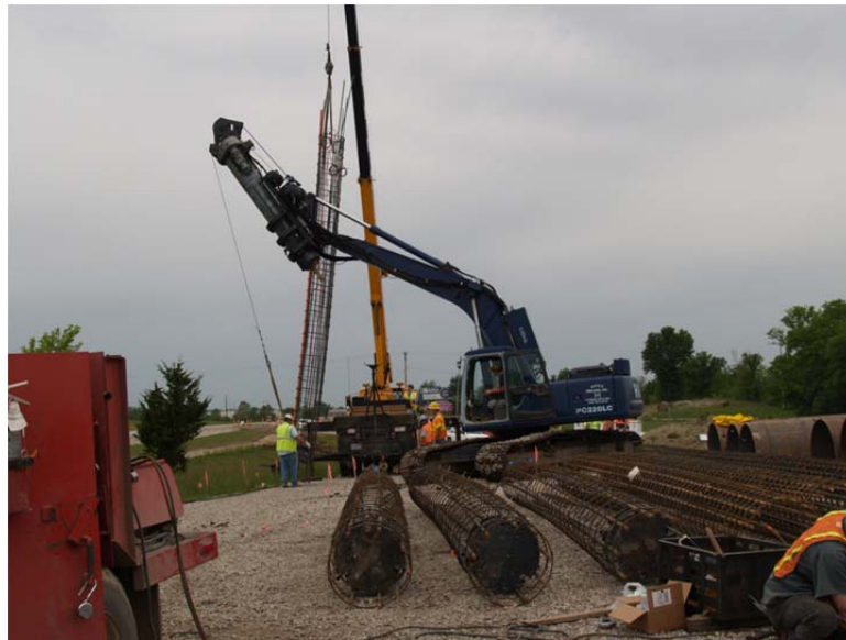
Figure 3.7- Reinforcement cage picked by the crane and drill rig.
