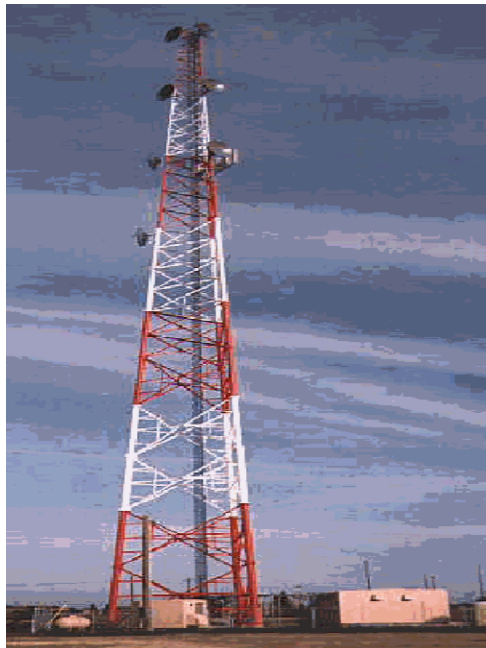
Figure 2.1. Example of a typical self-supporting (free standing) tower.
