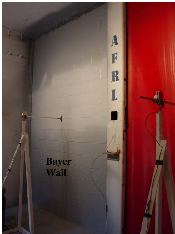
Figure 5.25 – CMU Wall with Bayer Polymer Retrofit
