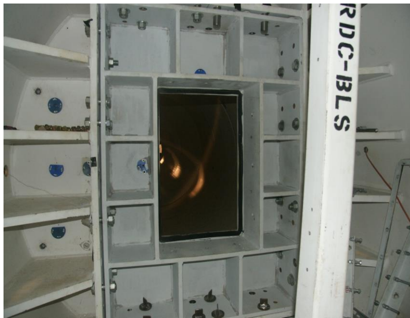
Figure 2.9 Glass panel installation inside the BLS
