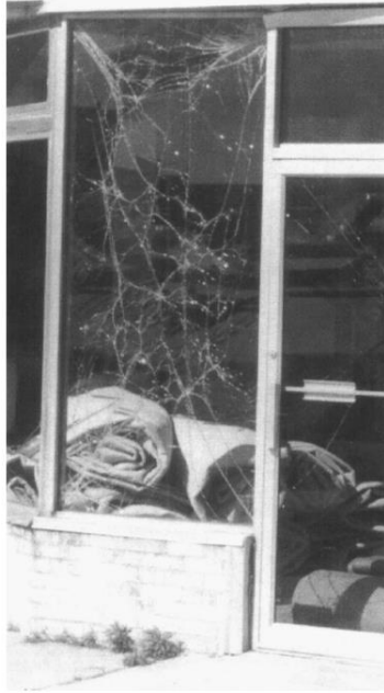
Figure 1.3 Laminated glass window and door fractured but remaining in frame in Oklahoma City bombing (Reprinted with permission from “Survey of window glass broken by Oklahoma City bomb on April 19, 1995, revised”, copyright belong to Glass Research and Testing Laboratory, Texas Tech University).
