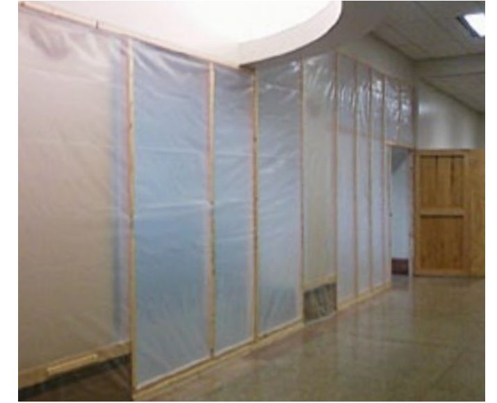
Dividers were erected around the circulation, reserve and interlibrary loan offices, which is where the fires were set.
