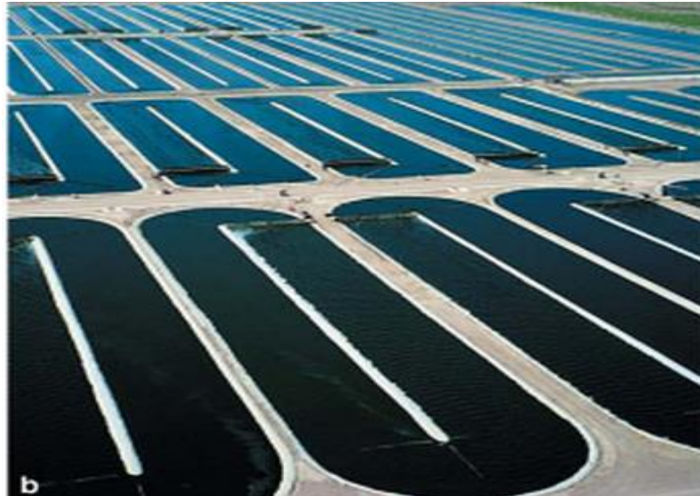
Figure 1.8 Image of an open pond system (Wen, 2014)
