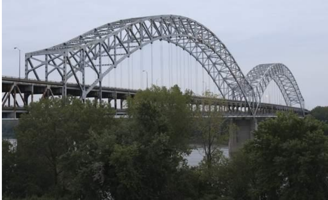
Figure 1-1: Sherman Minton Bridge (Stone and Green 2011)
