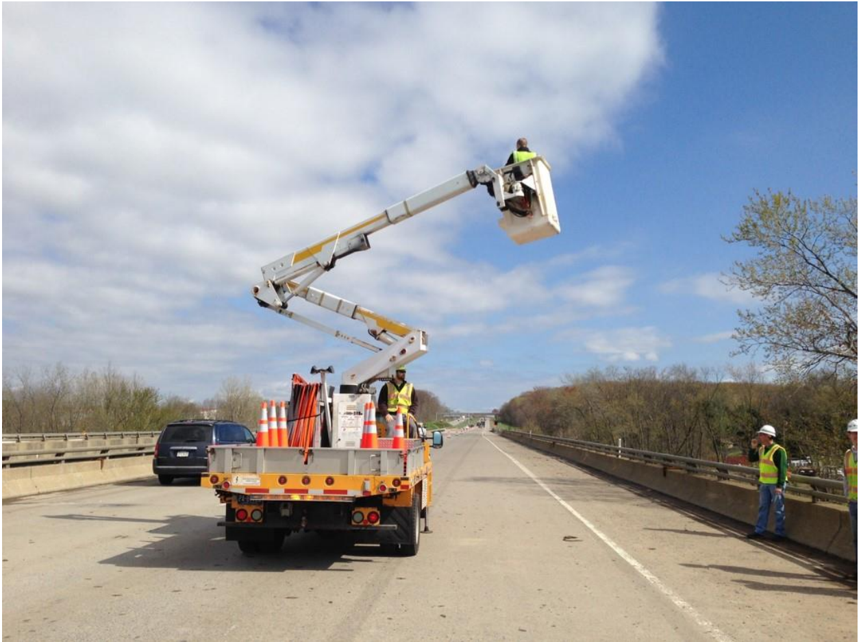
Figure 4-24: Boom truck utilized for imaging a bridge deck from an elevated location
