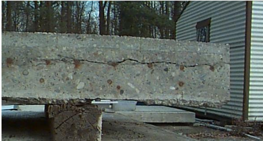
Figure 2-1: Delamination at the embedded steel level
