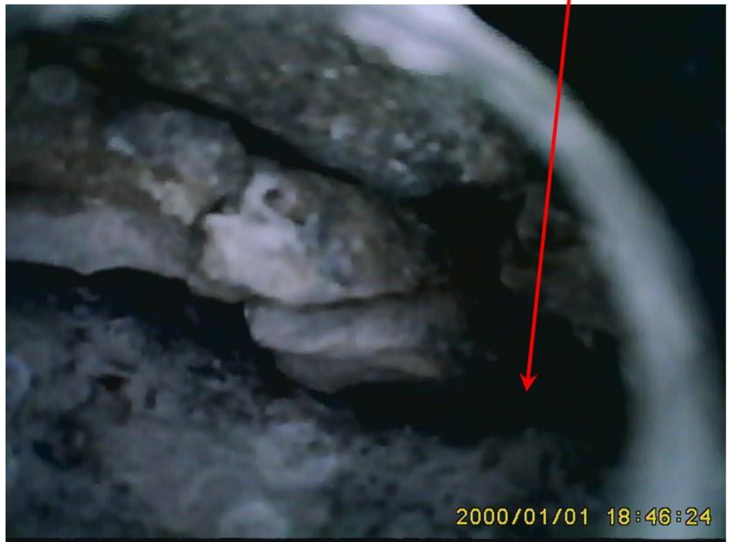
Figure 4-14: Borescope image of a deck delamination
