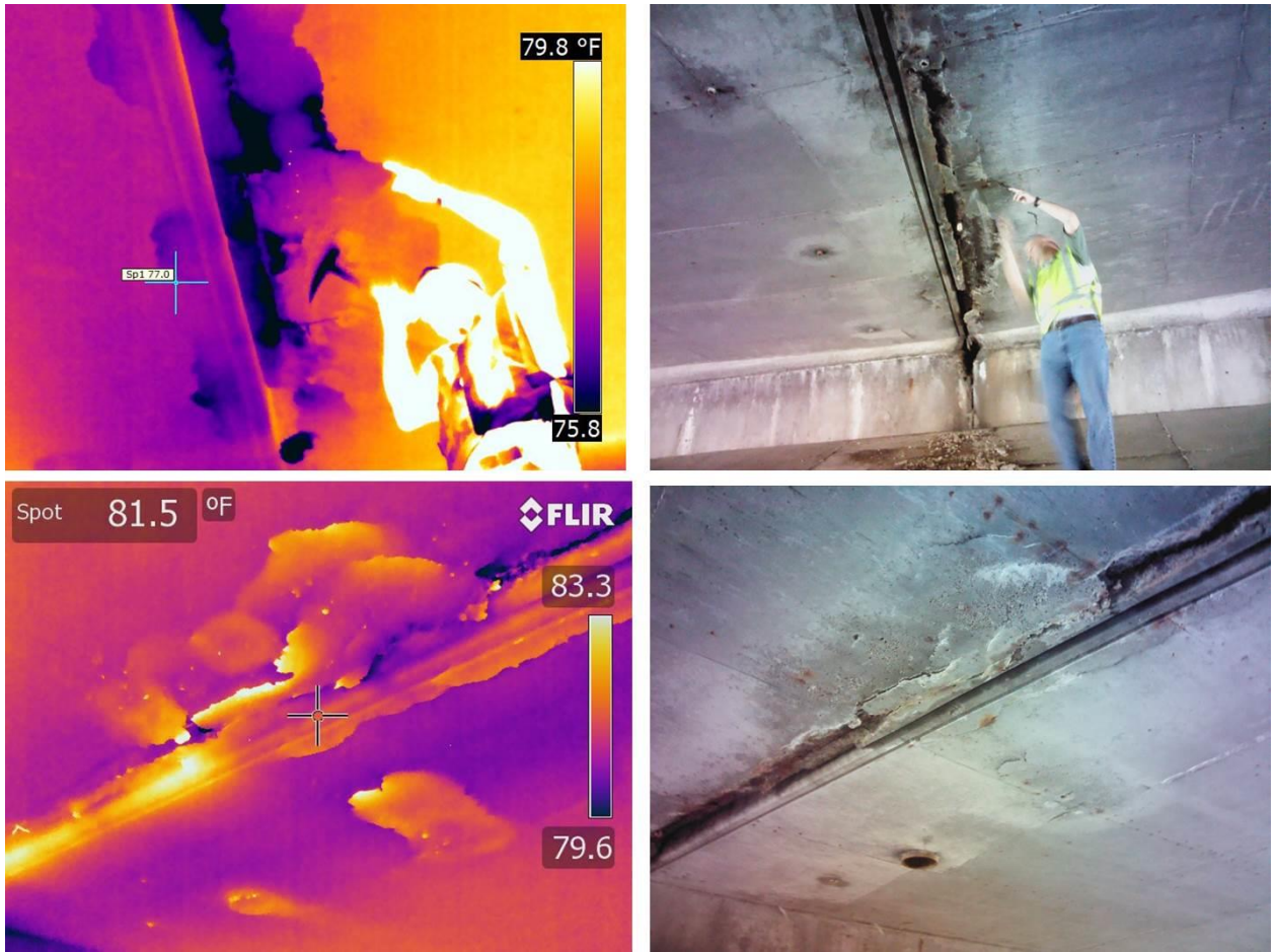
Figure 4-40: Thermal images showing damage along a longitudinal joint in a 159 ft wide slab bridge
