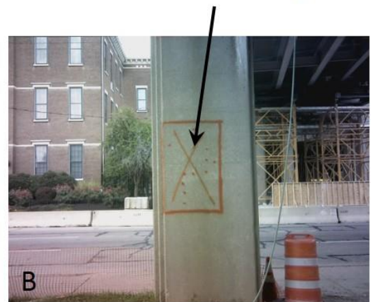
Figure 4-32: IR (A) and digital (B) images of hammer sounding results on a pier in Kentucky
