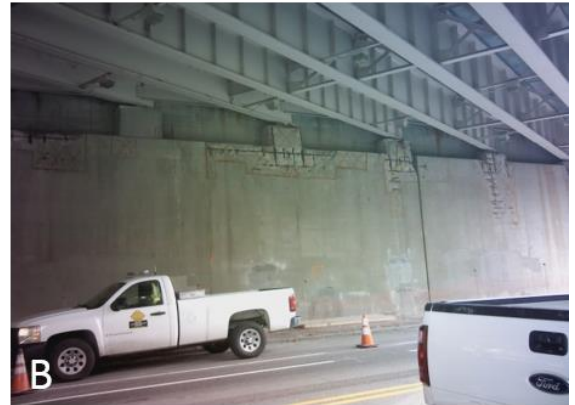
Figure 4-31: Thermal (A) and Digital (B) images of a delaminated abutment wall under I-265
