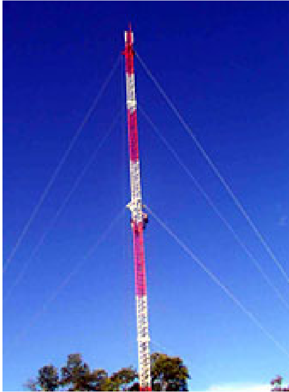
Figure 1.2 A guyed tower with four guyed layers.
