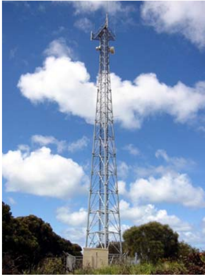
Figure 1.1 A self supporting telecommunication tower.
