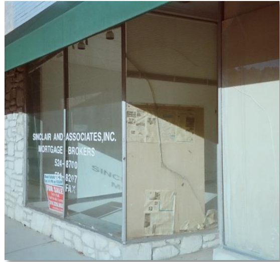
Figure 49. Vacant commercial building.
