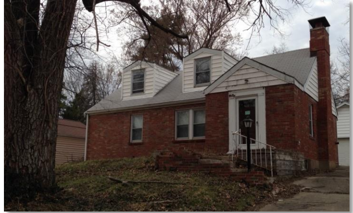
Figure 39. Abandoned home overlooking Jeske Park.
