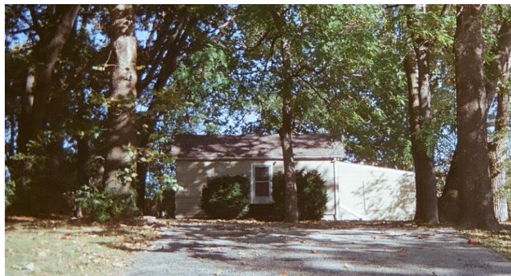
Figure 45. Abandoned home; painted plywood.
