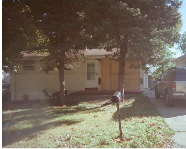
Figure 46. Abandoned home; neighbor parked in driveway.
