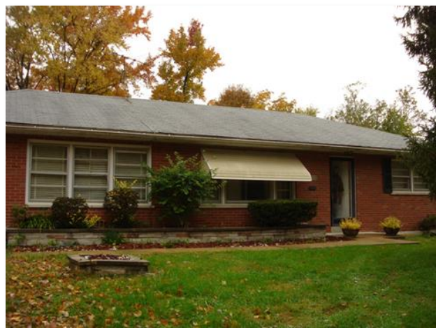
Figure 2. Example of brick house constructed Post-WWII.
