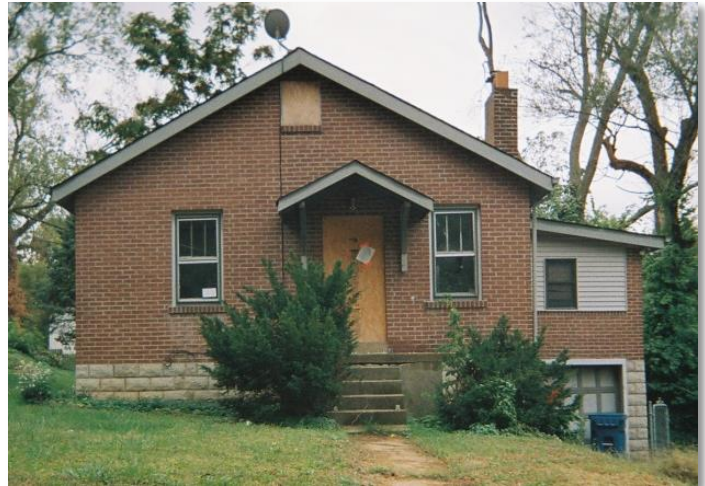
Figure 42. Abandoned, boarded up home.
