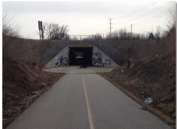
Figure 13. Artwork on tunnel.
