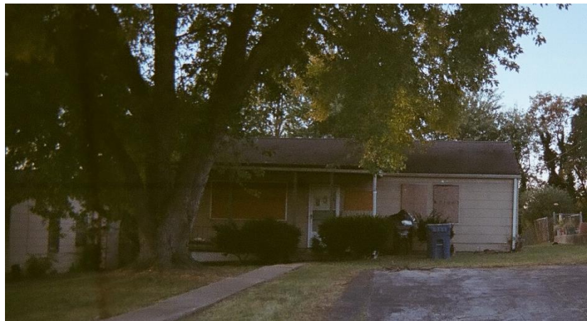
Figure 68. Boarded up; abandoned rental property.
