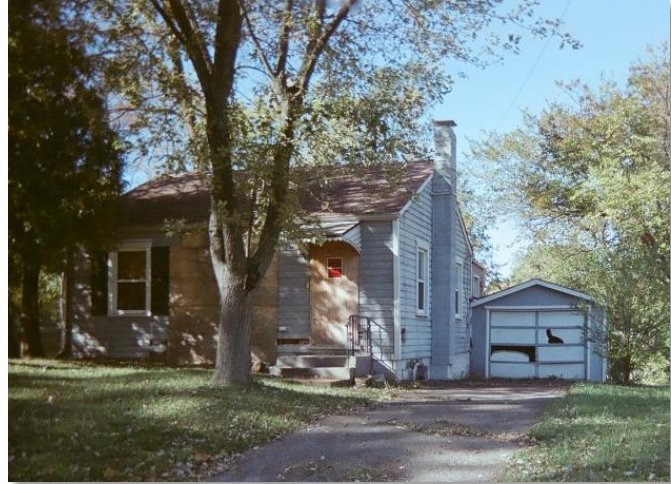
Figure 44. Abandoned home; plywood over doors and windows.
