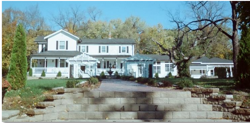
Figure 37. Remodeled historic home.
