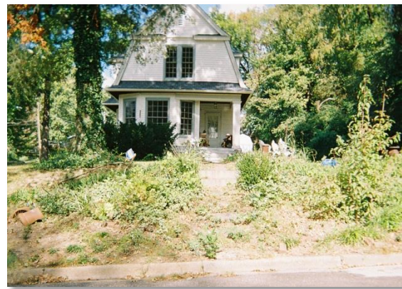
Figure 59. Home with overgrowth.
