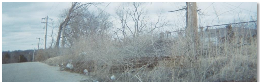
Figure 65. Overgrowth hanging into street.
