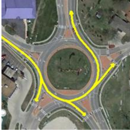
Figure 1.2.1 Roundabout intersection in Branson, MO, Business 65 and Branson Landing Blvd. (Google, 2014)
