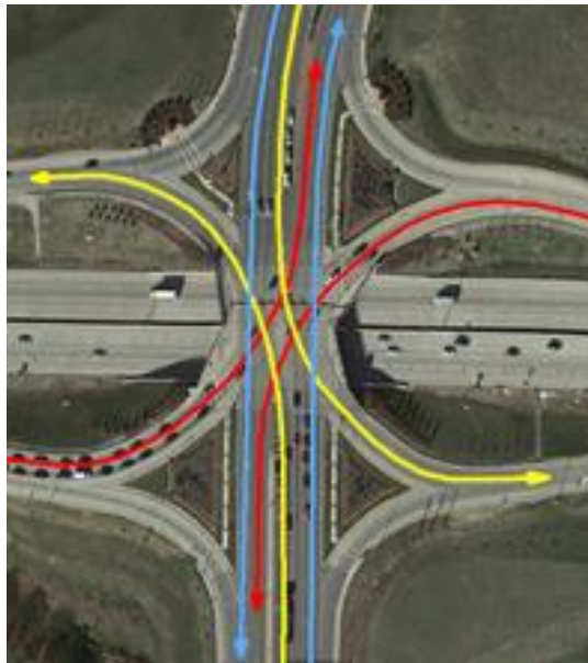
Figure 1.2.2 Single Point Urban Interchange (SPUI) in St. Louis, MO, I-64 and S. Kingshighway Blvd. (Google, 2014)
