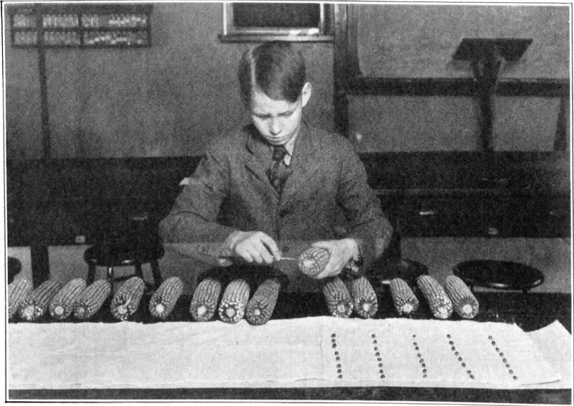
Fig. 2.—Removing the kernels and placing on rag-doll tester.
