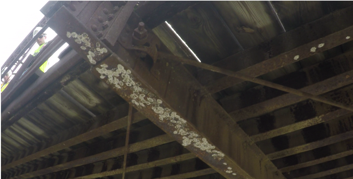
Figure 14: Camera footage from tethered aircraft during substructure inspection.
