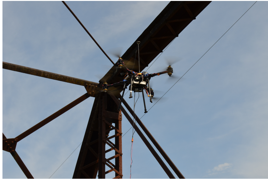
Figure 13: Tethered aircraft during superstructure inspection.
