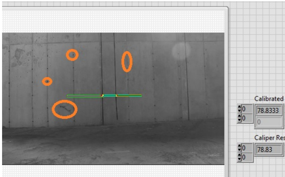
Figure 26: Parking structure wall imperfections.
