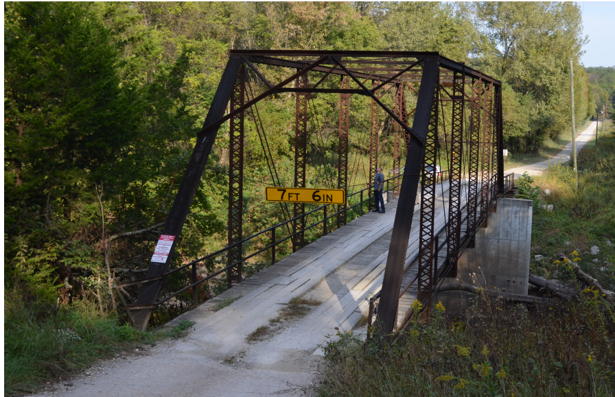
Figure 12: Fracture-critical, structurally deficient Boone County bridge.
