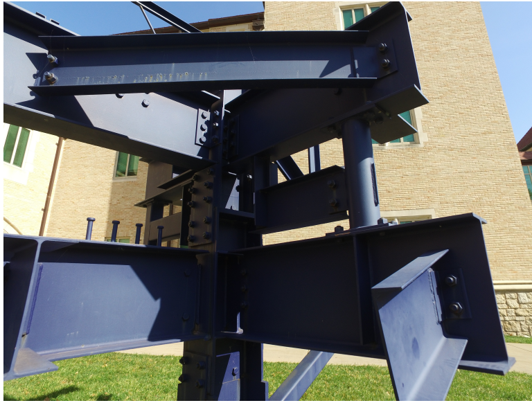
Figure 16: Steel construction with manual underexposure.
