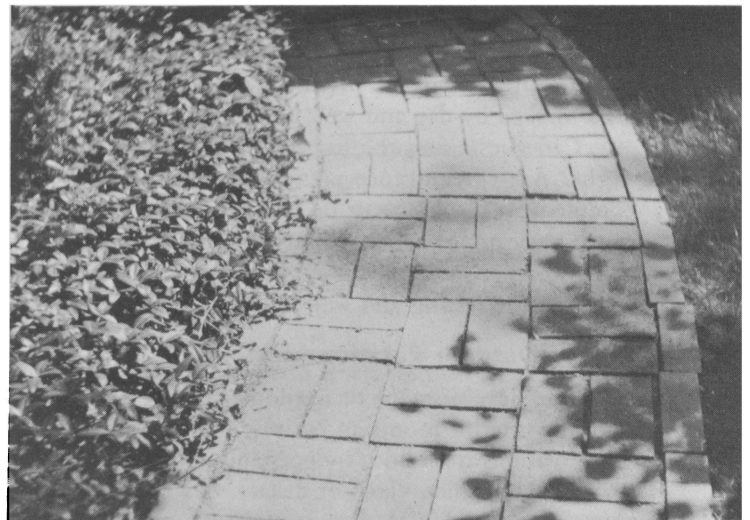
This brick walk laid in a basket weave pattern has ample width for two people to walk side by side.
