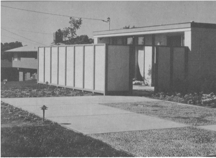
A baffle around a bedroom patio stops wind and screens view from neighboring houses.
