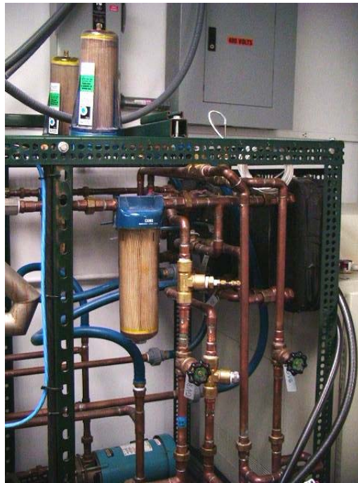
Fig. 9. Air handler conditioning loop Flat Plate® heat exchangers.
