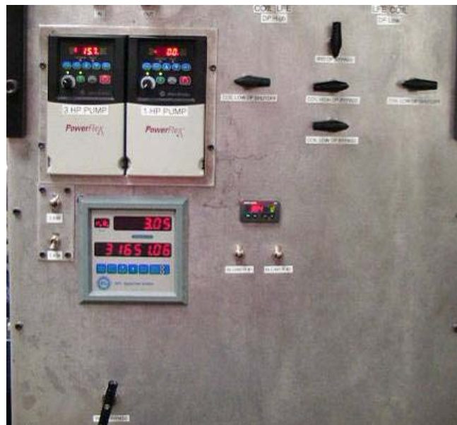
Fig. C4. Wind tunnel control panel.
