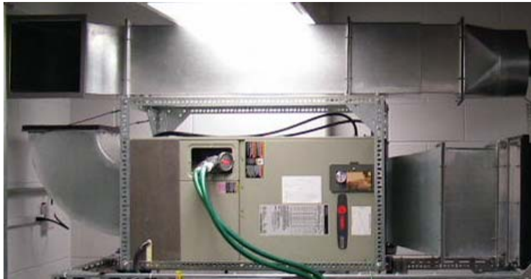
Fig. 4. Original air handler used in early Unit Cell tests.
