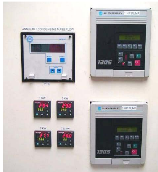
Fig. C6. Picture of Air Handler Conditioning Loop 1 control panel.
