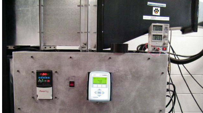
Fig. C5. Air handler control panel.
