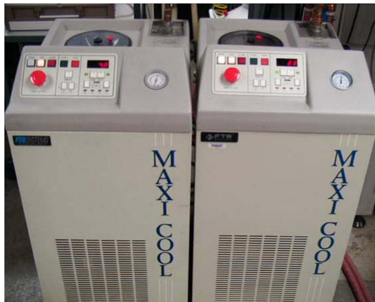
Fig. 10. Maxi-Cool chillers used for supplement heating and cooling for Air Handler Conditioning Loop and Unit Cell Liquid Loop.
