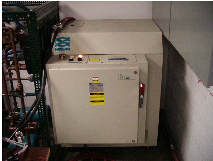
Fig. 11. HX540 NESLAB® chiller used for cooling for Air Handler Conditioning Loop.
