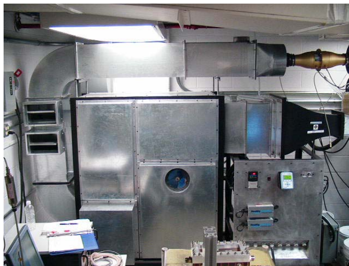
Fig. 5. Current air handler.
