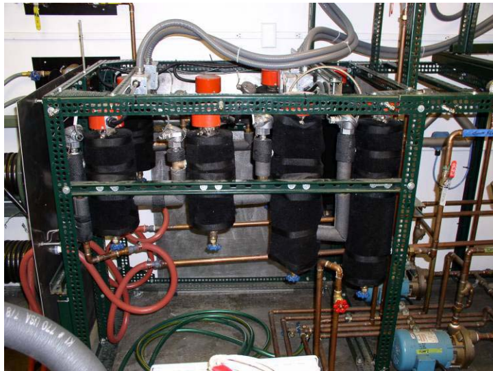
Fig. 12. Air handler conditioning loop heater section. Watlow® resistive heaters 1 kW, 3kW, 6kW, and 7.5kW.
