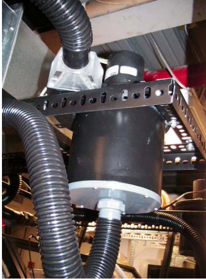
Fig. 20. Air blower for temperature measurement
