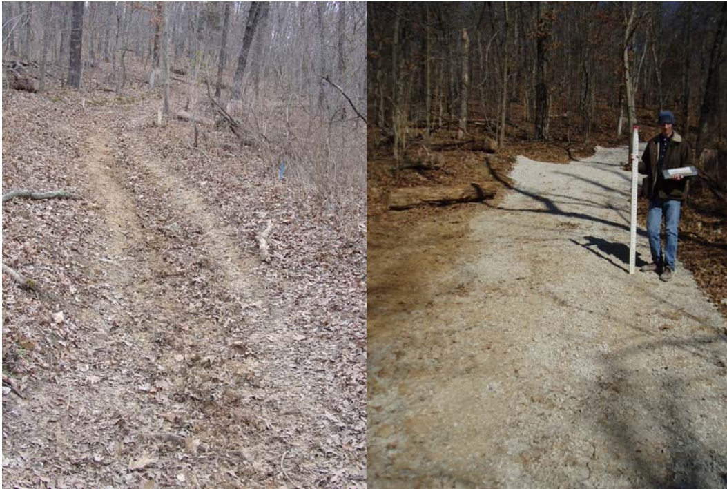
Figure 4-9. Segments 16 through 18 Before and After Treatment.
