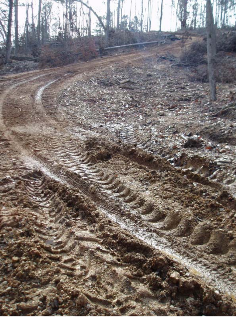
Figure 4-19. Ruts and Muddiness Observed on Sections 21 and 22.
