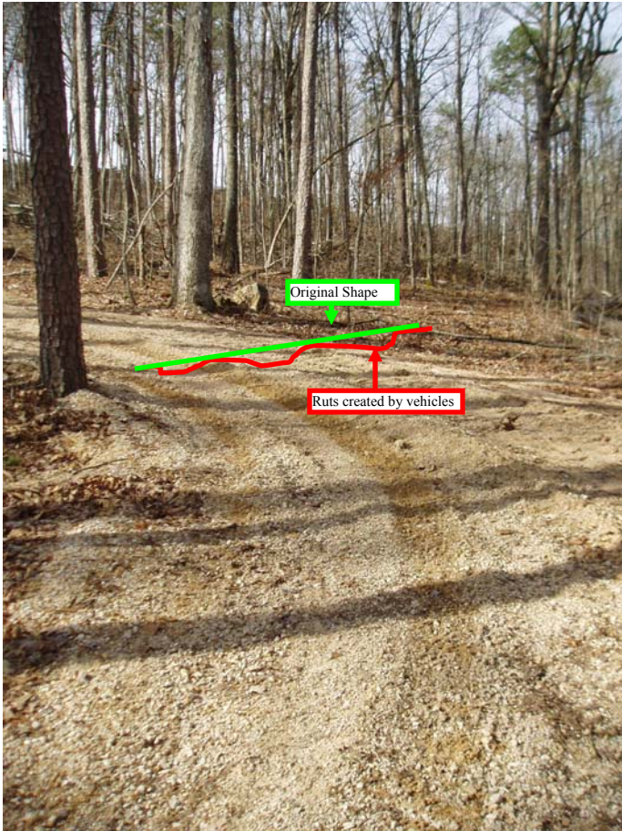
Figure 4-18. Ruts from Wheeled Vehicles on Sharp Turns.
