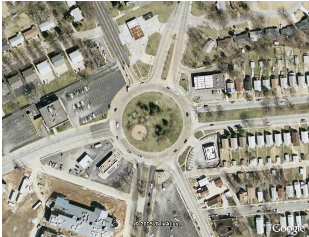
Figure 7: Ariel photograph of the Halls Ferry Circle (Google, 2007)
