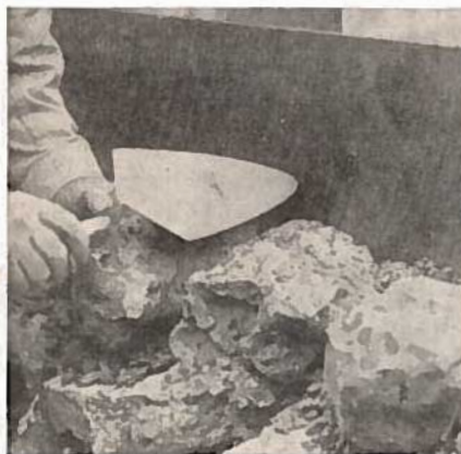
Fig. 7A.—Gauging thickness of wall. Trowel is used to measure distance from face of form to outer face of wall.
