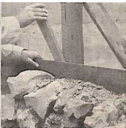
Fig. 4B.—Removing strip after nail has been pulled. This allows form to be taken off and raised.
