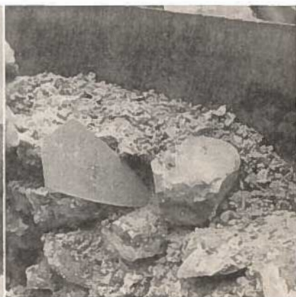
Fig. 8B.—Raking out the joints. After mortar has hardened somewhat the surplus is raked off the face of the stone.
