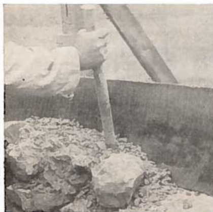
Fig. 8A.—Tamping concrete. Use short broom handle or similar tamper to insure compact concrete.
