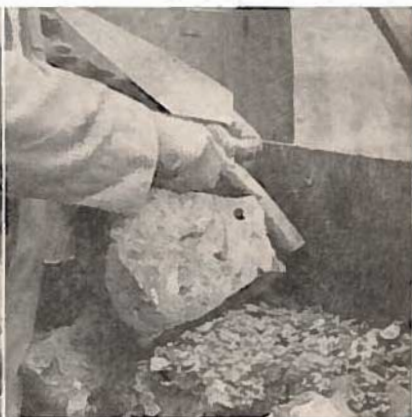
Fig. 7B.—Using handle of trowel to insure space for mortar between stone and form. Rocks should not be jammed against form.
