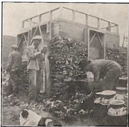
Fig. 3.—Window frames and door frames are tacked on outside of forms.
