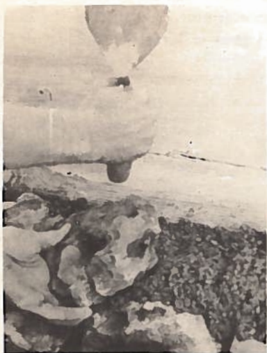
Fig. 12.—Tamping rock firmly into place.
