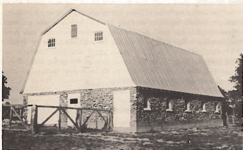
Fig. 8.—General purpose barn built of cobblestone.
