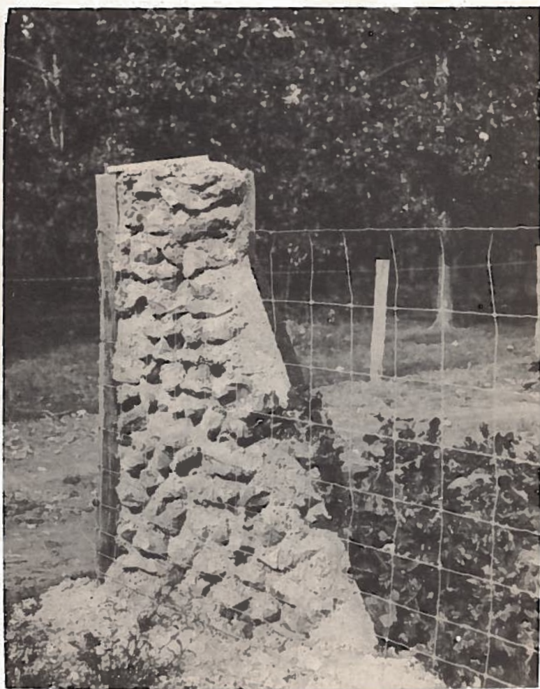
Fig. 17. —Substantial and non-rotting corner post built with field rocks found on the farm.
