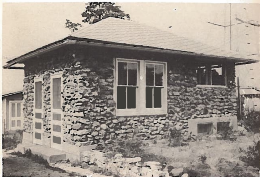
Fig. 16.—Two Room Milk House. Rock construction makes a very sanitary milk house.
