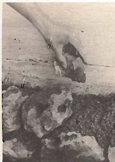
Fig. 14.—Working small rocks into mortar.
