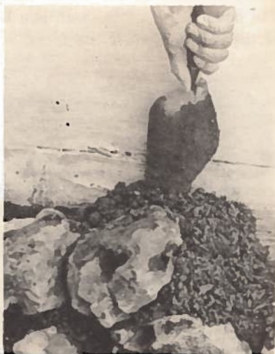
Fig. 13.—Spading concrete into place.
