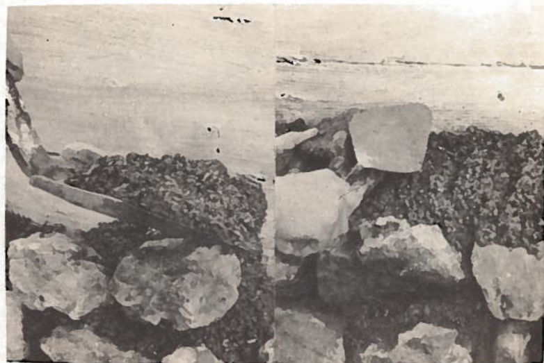
Fig. 10.—Preparing mortar bed. Fig. 11.—Placing rock by measuring out from form.
