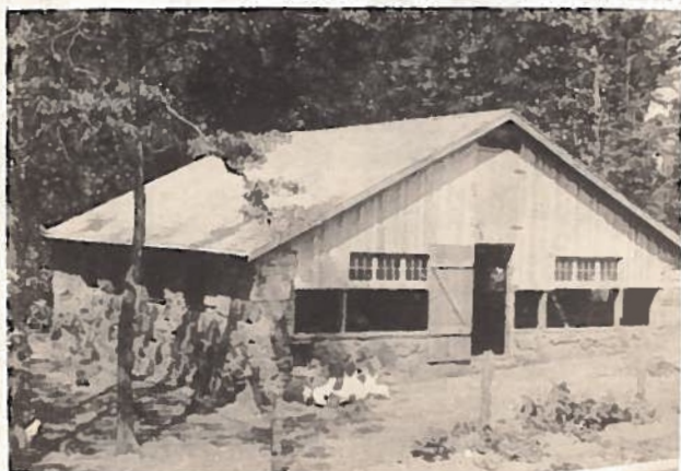
Fig. 9.—Missouri type 30x30 Poultry House built of flat rocks. Rock poultry houses have proved very satisfactory in Missouri.
