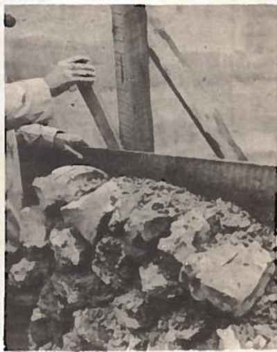
Fig. 5B.—Removing strip after nail has been pulled. This allows form to be taken off and raised.
