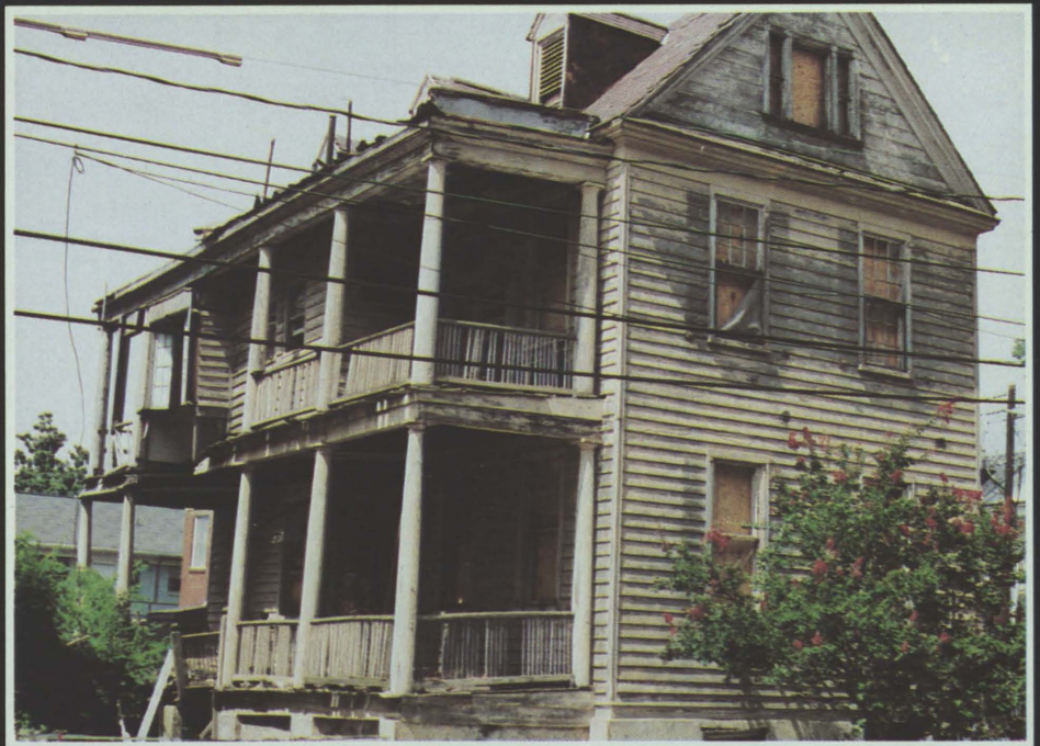
Remnants of homes in Charleston, S.C. post Hurricane Hugo.
