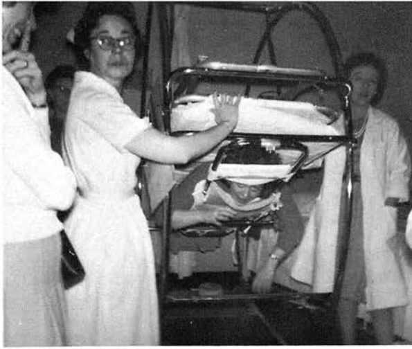
"The electricity's off?"
