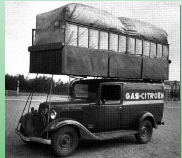
NG vehicle ~1930 (France) with balloon tank on roof
