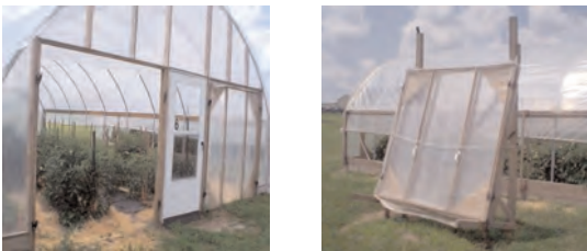
Figure 9. End wall panels can be removed (left) and stored (right) during the summer.
