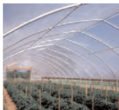
Figure 4. Purlins can number from one to four on a high tunnel.
