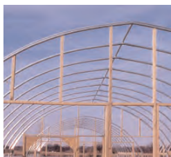
Figure 4. Purlins can number from one to four on a high tunnel.
