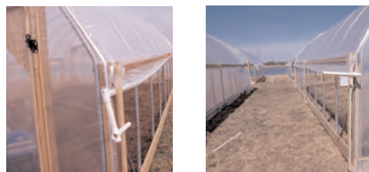
Figure 11. A \frac{3}{4} -inch PVC t-handle (left) rolls the sidewall vents up (open) or down (closed).
