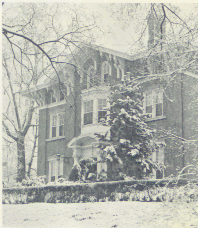
The Chancellor's Residence is the oldest building on campus, with the main section built in 1867.
