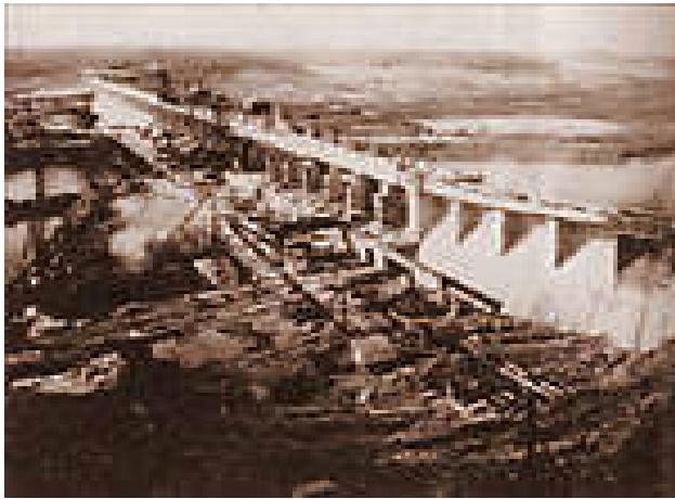
Bagnell Dam During Construction. 11
