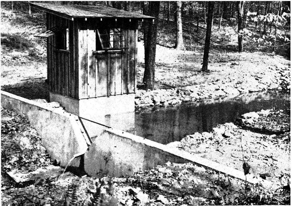
Fig. 6—Gaging station with modified 90° V-notch weir on Gum Springs Watershed.
