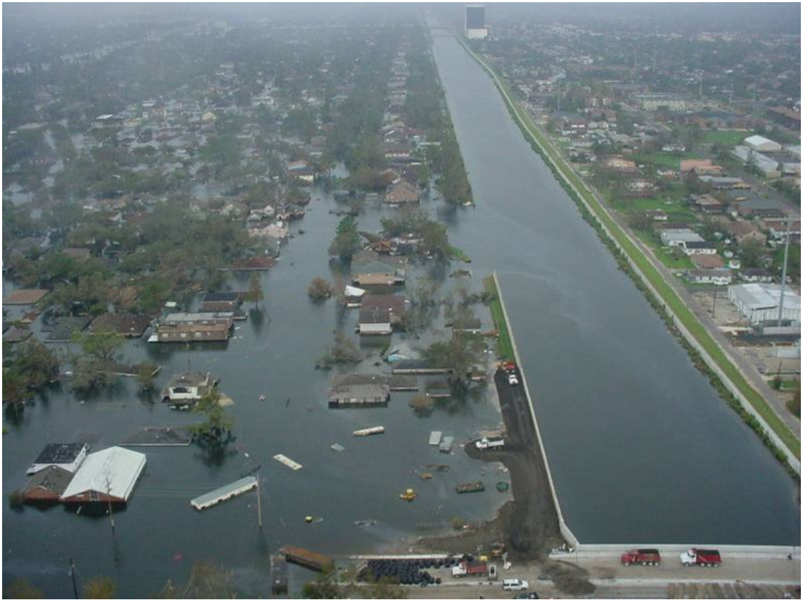
Figure 6: Canal levee failure in New Orleans, LA Example of man-made flood protection measure failure increasing damage Shown is the 17th Street canal that failed during hurricane Katrina in 2005
