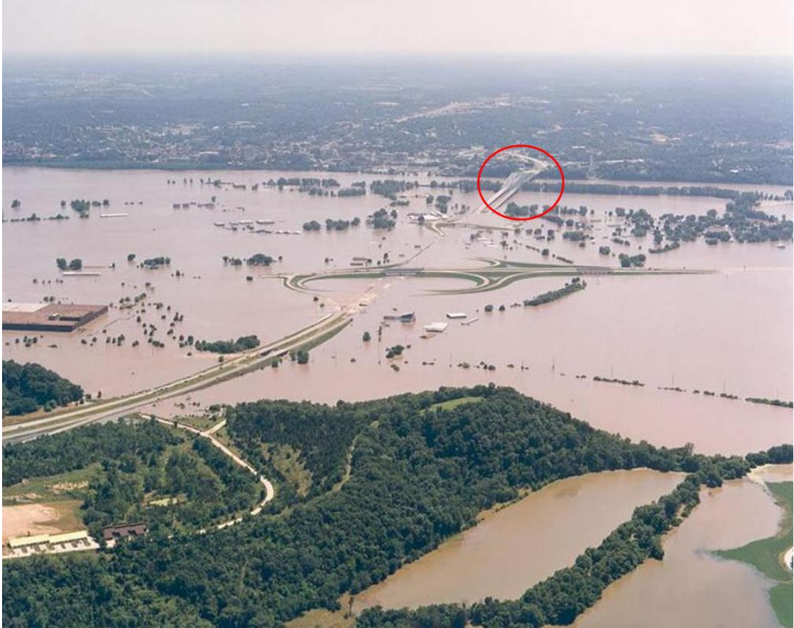
Figure 2: Highway 54 / 63 interchange north of Jefferson City, MO Looking south across flooding into Jefferson City, MO on July 30, 1993 Seen at the top of the floodplain is the bridge spanning the normal river channel (Photograph from Missouri Highway and Transportation Department)
