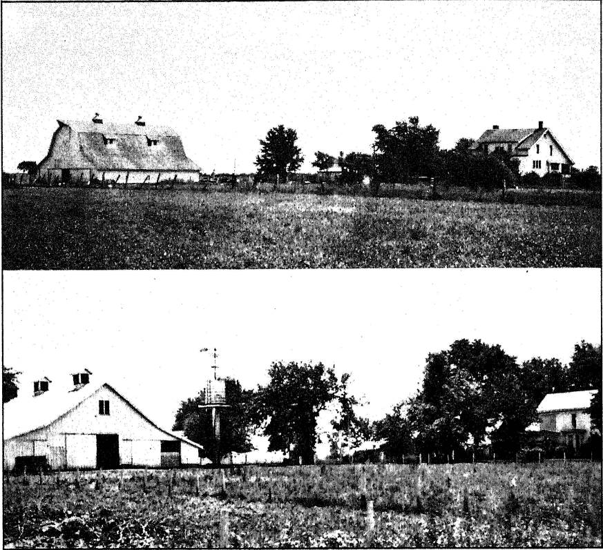
Figure 14.—These pictures illustrate farm buildings in Class A.
