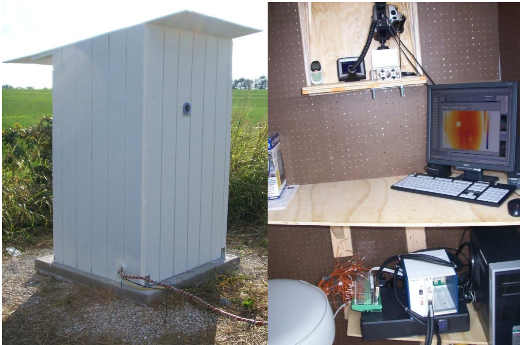
Figure 3.10 : Data House with inside layout.
