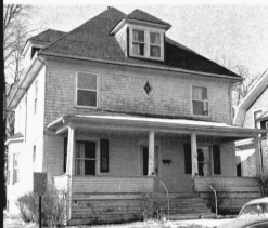
705 Gentry Office Space
