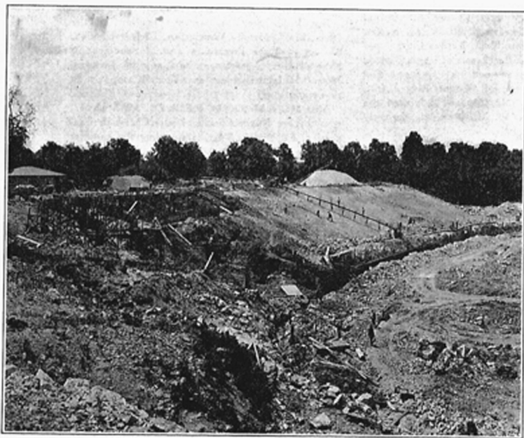
View showing pouring of concrete for east bleachers now well under way. The west bleachers have been completed. (See the advertising of H. H. Carrothers, Stadium contractor.)
