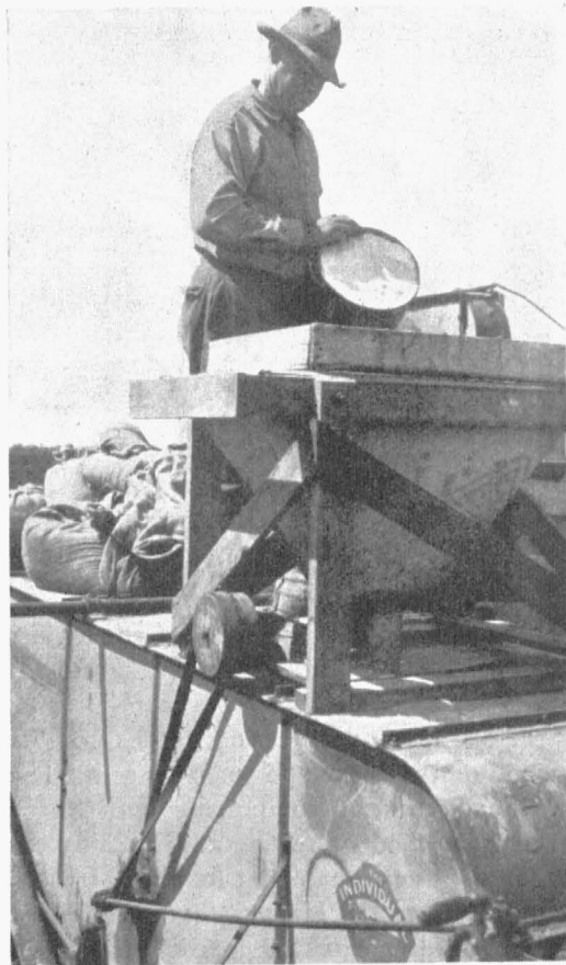
Fig. 6.—A simple apparatus for putting the reagent into thresher for artificial manure production. (Designed by E. M. Poirot, Golden City, Missouri.)
