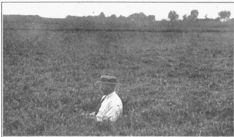
Fig. 12.—Land reclaimed by soil-saving dam. About a four-foot fill has been secured. The man is standing in the vertical intake pipe of the original dam.
