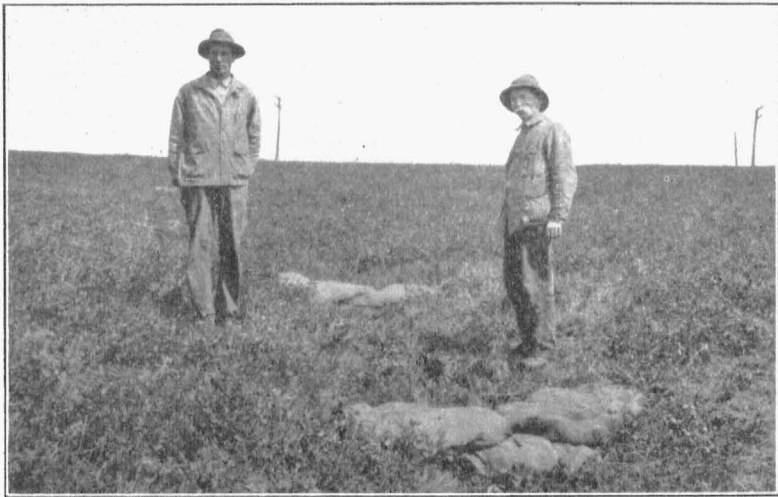
Fig. 8.—Bags of bluegrass sod placed in a clover field to stop gullying on farm of J. O. Erhart, Cole County, Mo. Mr. Erhart, the originator of this method, stands at the right.
