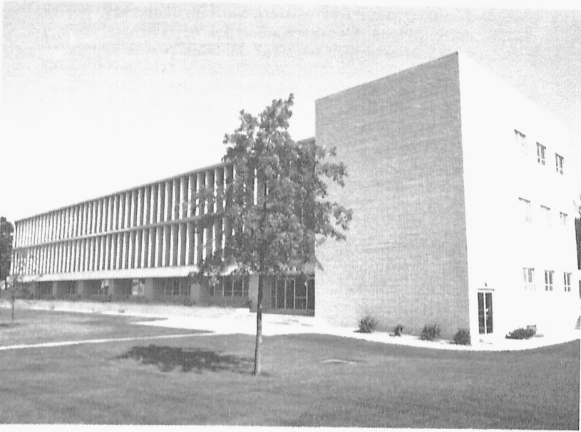
Electrical Engineering Building.
