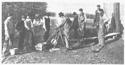
Testing steam drill, Mining and Metallurgical Laboratory, 1897-1898.
