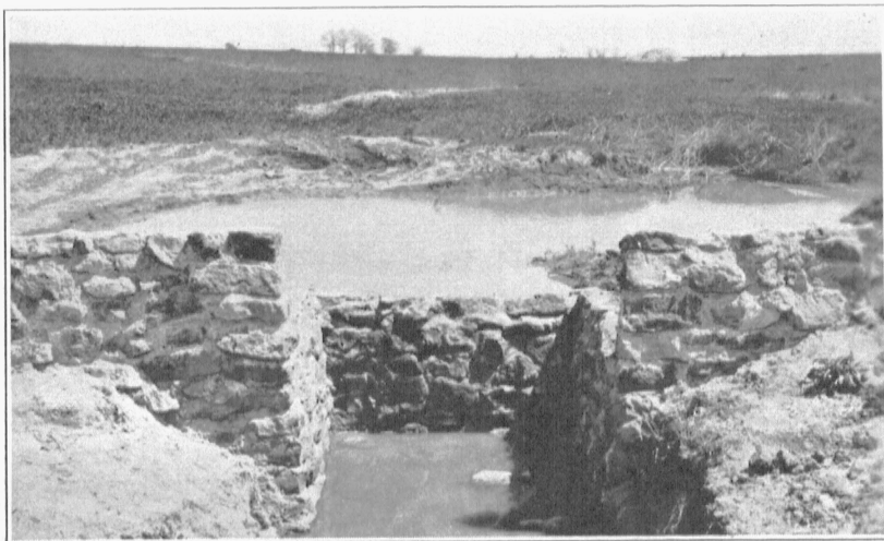
This rubble-masonry soil saving dam on the R. W. Lacy farm in Cooper county was built by the members of the leaders' training school.
