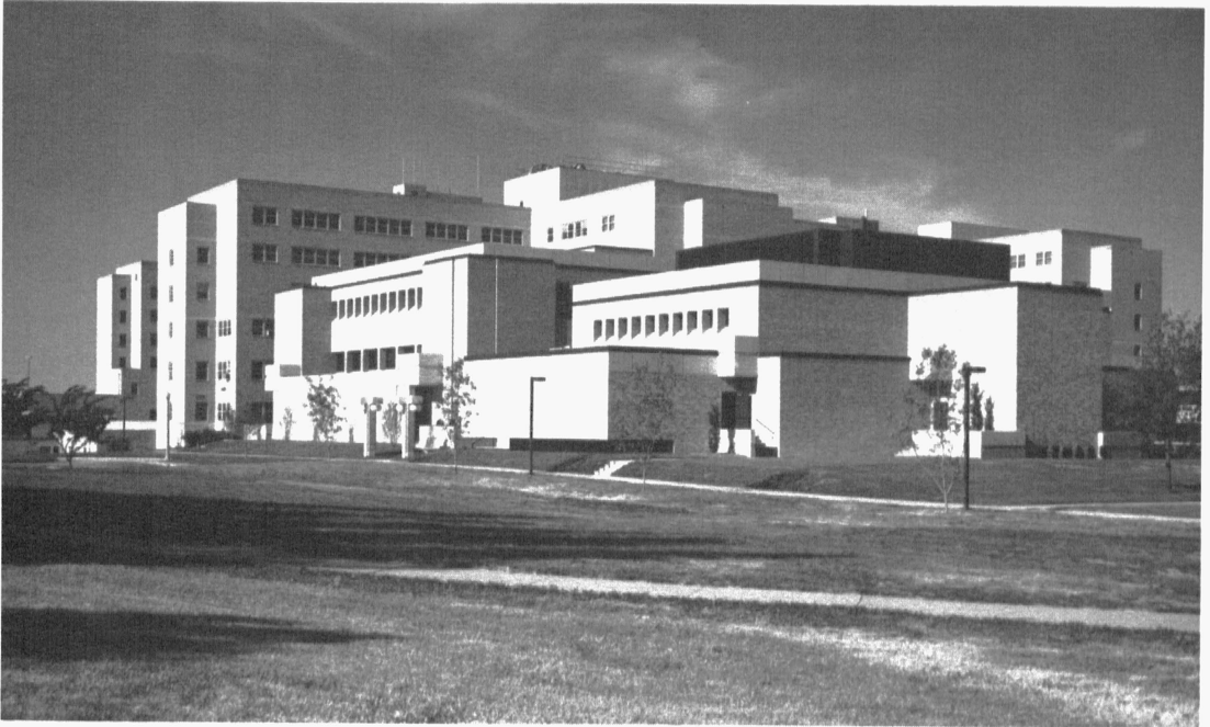
The new building was dedicated in 1980.
