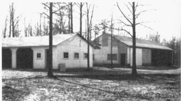
A four-stall garage (left) and a repair shop and equipment building to adequately service and protect automotive and other equipment were built at the University Forest during the period 1958 to 1961.
