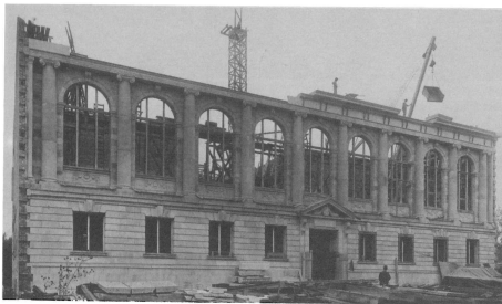
The Main Library under construction, 1914.
