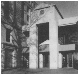
West entrance to the new addition.
