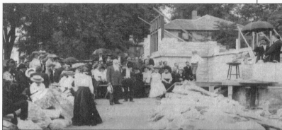
The founders of the Missouri School of Religion translated vision into concrete form when they began construction of Lowry Hall in 1904.
