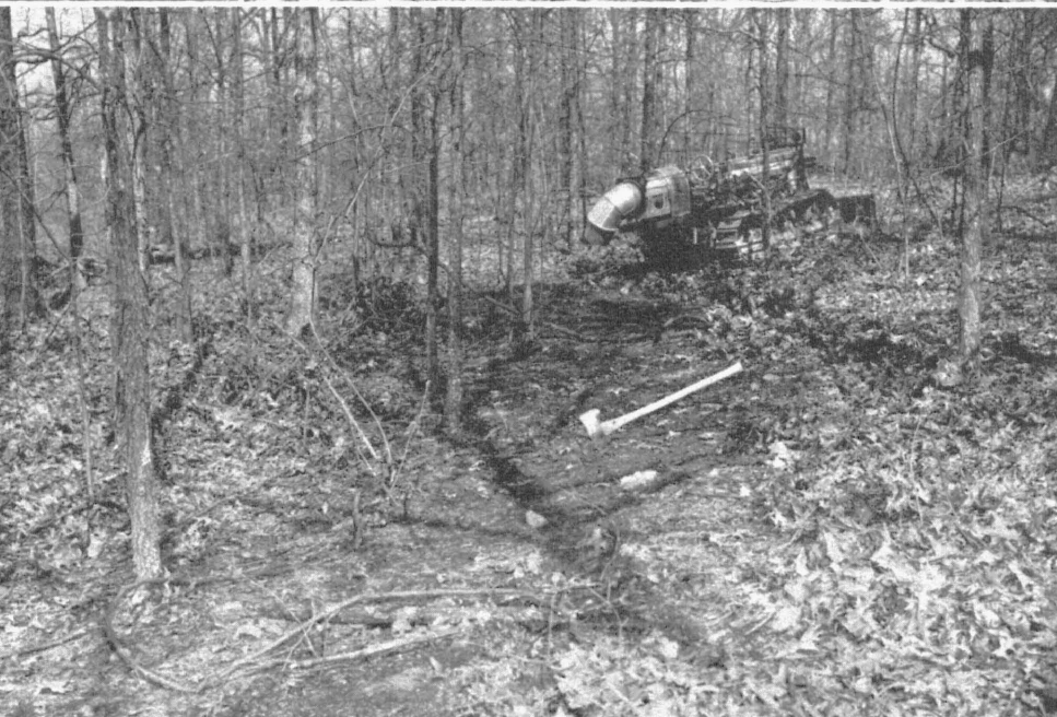
Completed fire line more than six feet wide across the area.
